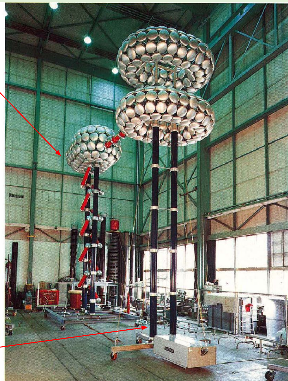
DC voltage test set 2000 kV, 10 mA for testing power cables, including a HV measuring resistor and automatic grounding system (foreground)
