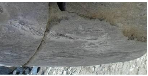
Protect the adapter weldings
