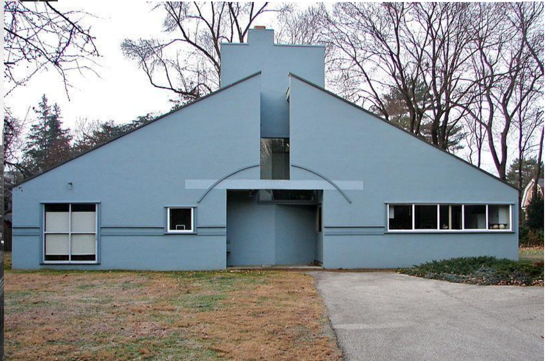
R. Venturi, Vanna Venturi House, Philadelphia, 1962-64
