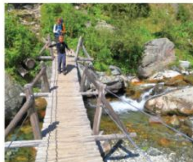
3 over the bridge
