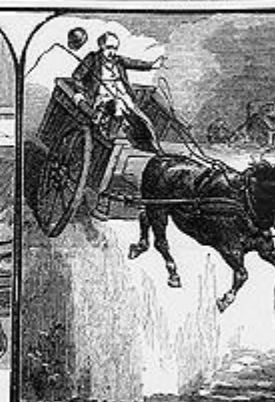
GREAT FALL OVER AN EMBANKMENT BIRKENHEAD
