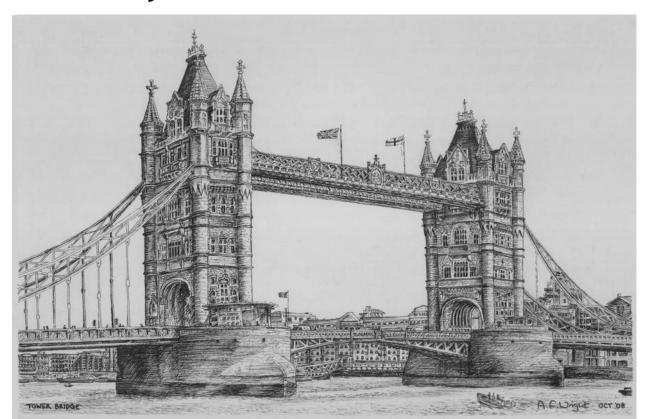
• Even today Tower Bridge regulates a large part of the impressive traffic of the Port of London. Due to a special mechanism, the main traffic-way consisting of two parts fixed to two hinges at the ends can be lifted up. In this way, the entrance and departure of extremely large vessels is possible, and it allows them to reach the Pool of London.
