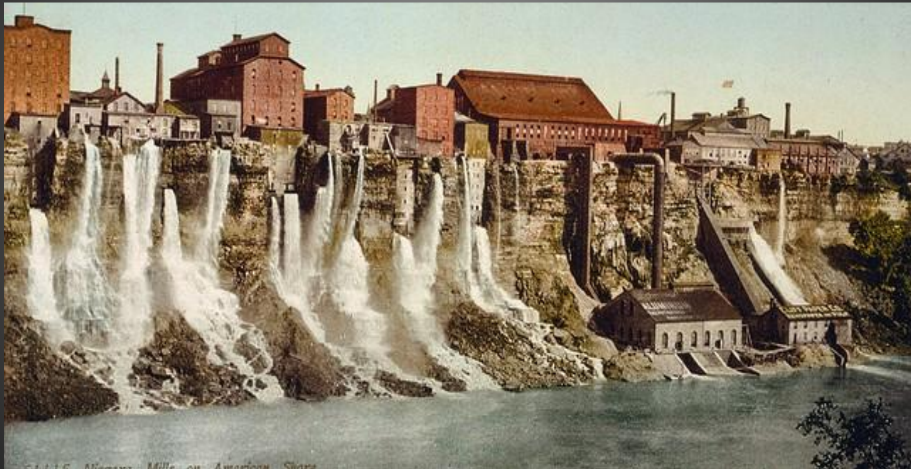
Fig. 1.5. Niagara Mills on American Side
