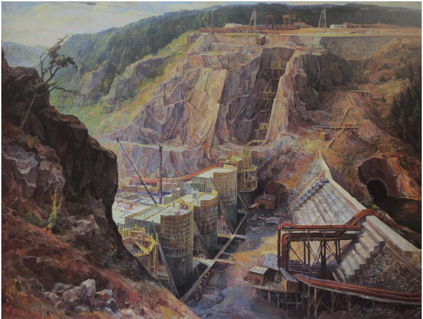
F. Bílek, Building of Dam Slapy, 1958
