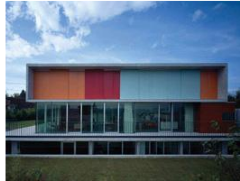
Private house in Basel (Switzerland), 2006
