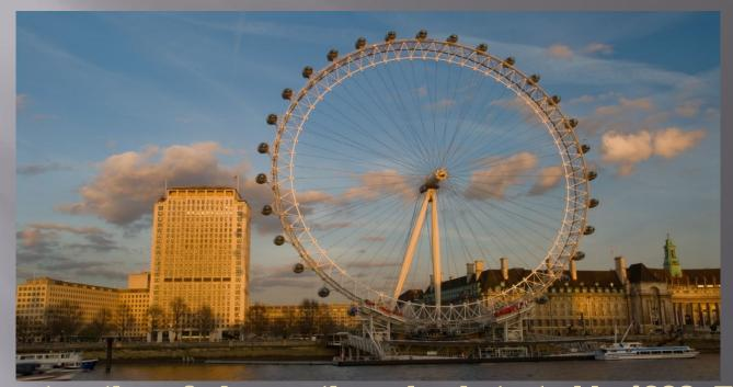
**Construction of observation wheel started in 1998.** The wheel was designed by architects David Marks and Julia Barfield. The wheel was constructed from segments that are transported up the Thames on barges and assembled on special platforms on the river. When the wheel was finished, it was raised to a vertical position using a special system of 2 degrees per hour until it reached 65 degrees. The total weight of steel in the "Eye" is 1700 tons.
