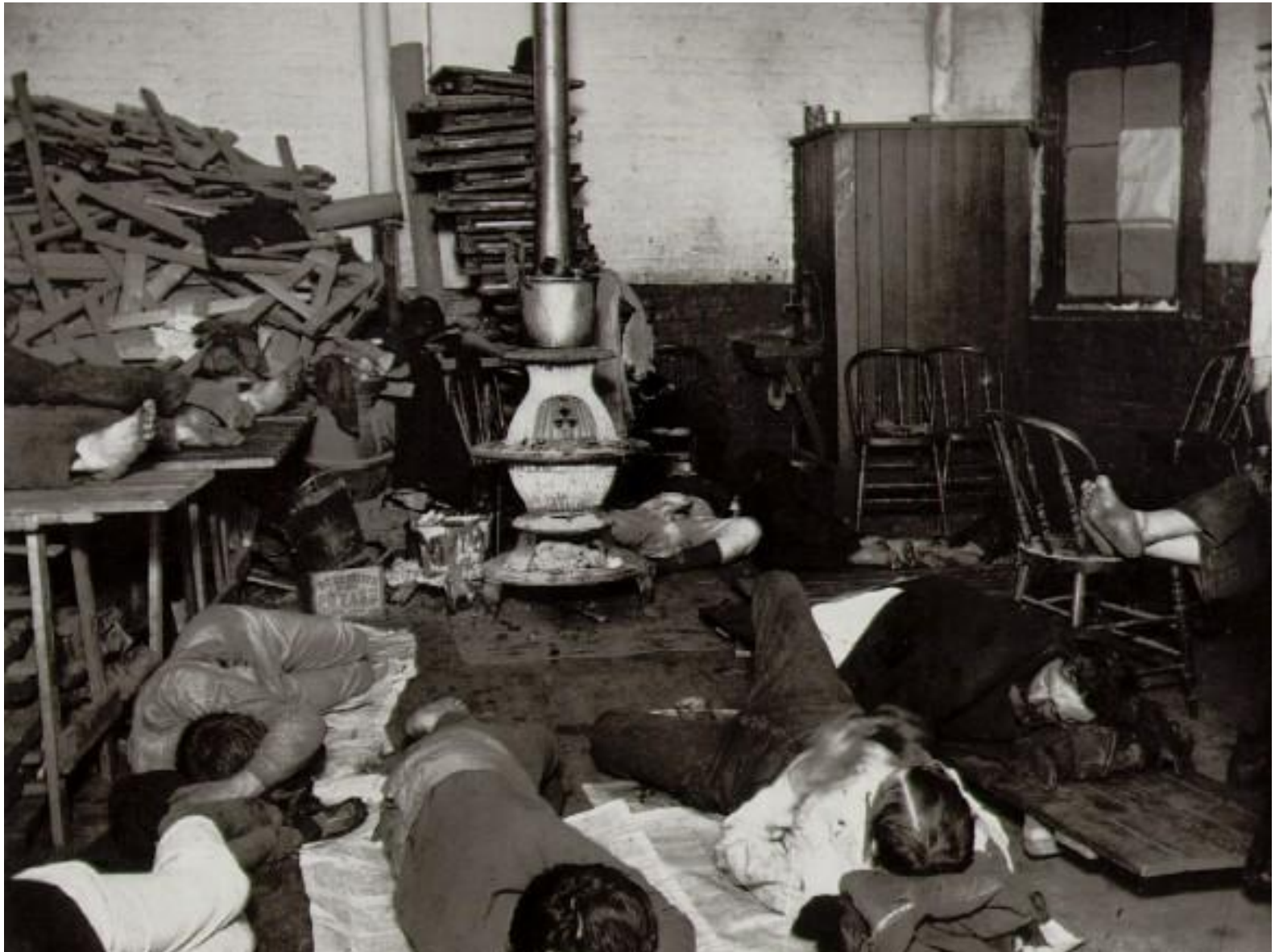
Men's Lodging Room in the West 47th Street Station.
