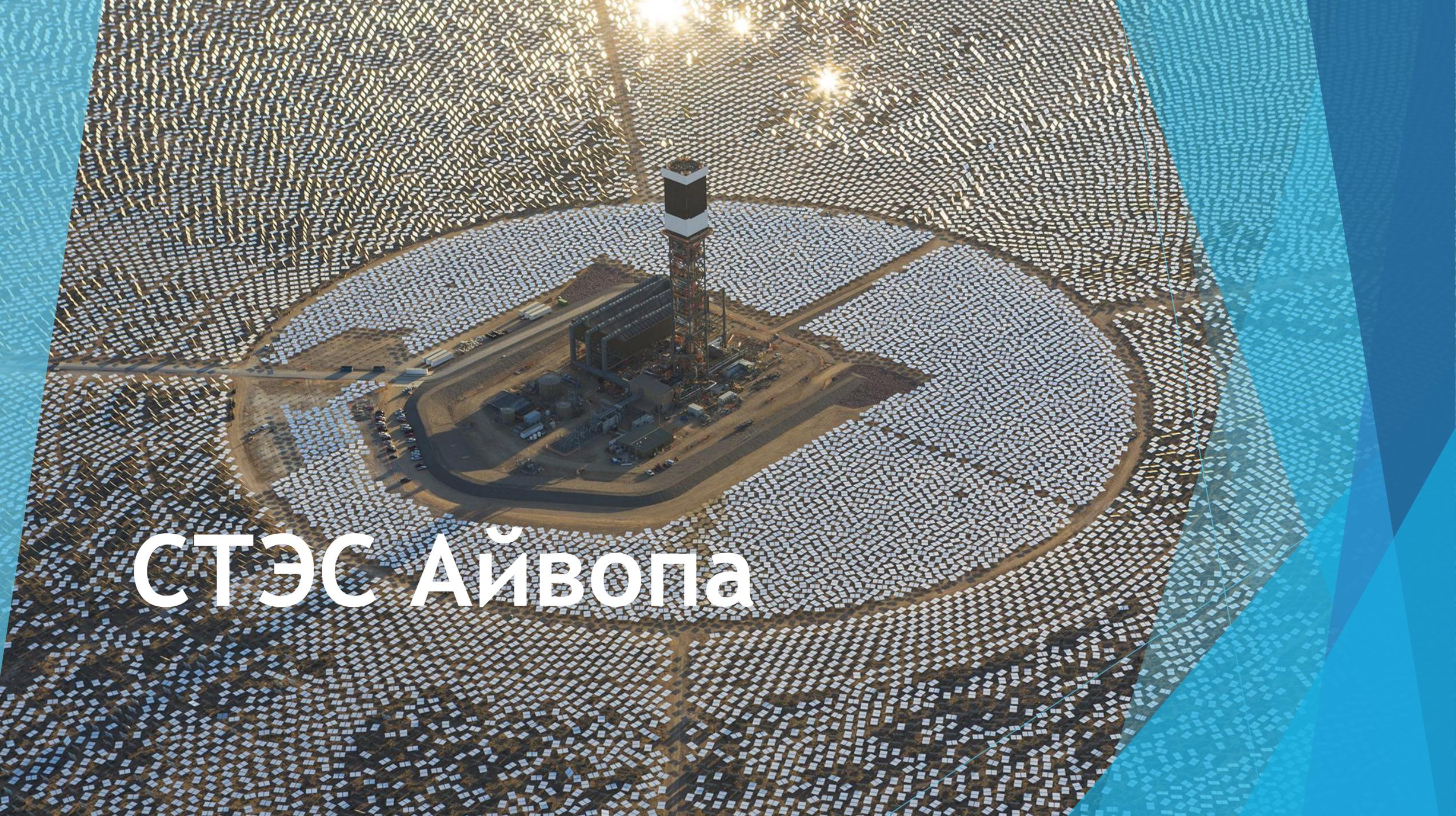
An aerial photograph of a solar power plant, specifically a Concentrated Solar Power (CSP) plant. The central feature is a tall, slender receiver tower (receptor) with a black and white top section. Surrounding the tower is a vast field of heliostats (mirrors) that reflect sunlight onto the tower. The plant is situated in a desert-like environment. The image is framed by a blue geometric overlay on the right side. The text "СТЭС Айвопа" is overlaid in white at the bottom left.
