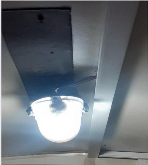
A photograph showing a white cable running along a metal beam in a ceiling or underfloor space. The cable is not secured in a cable tray or conduit, which is a violation of electrical safety standards. |
