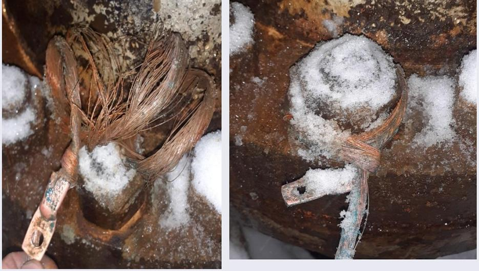
Two side-by-side photographs showing severe corrosion of electrical components. The left photo shows a bundle of copper wires and a terminal block heavily encrusted with white, crystalline deposits. The right photo shows a similar component, possibly a terminal or a small transformer, also completely covered in the same white deposits, indicating a lack of proper grounding and maintenance. |
