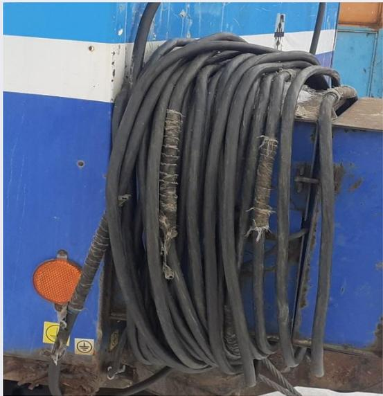
A photograph showing a bundle of thick, grey power cables. The cables are bundled together and appear to be in poor condition, with some fraying and damage visible at the ends. They are connected to a blue metal structure, possibly part of a power station or transformer. A yellow warning sign with a lightning bolt symbol is visible on the blue structure near the cables. |
