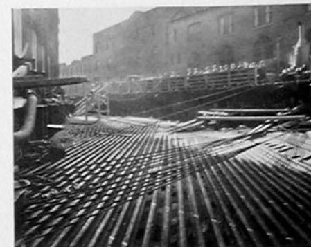
FIGURE 15. Pulling cables, trackage and arrangements for public to view operations.
