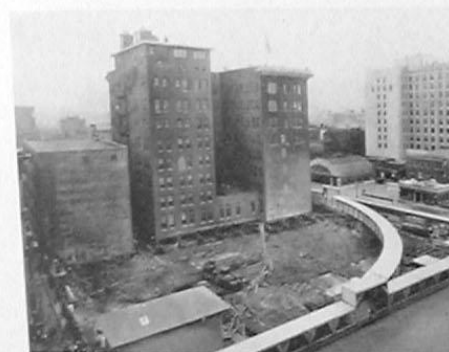
FIGURE 14. On the afternoon of November 12 the building move had been completed.
