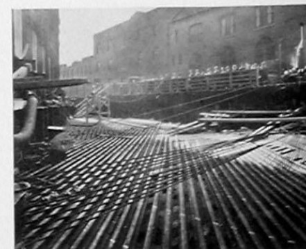
FIGURE 15. Pulling cables, trackage and arrangements for public to view operations.
