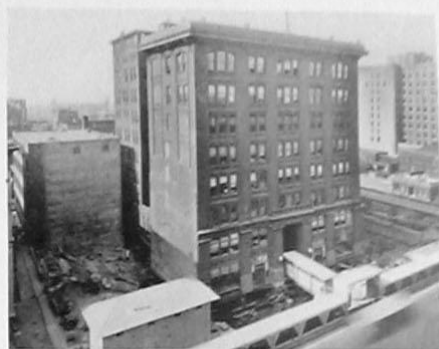
FIGURE 5. On October 18 the structure had reached the end of the straight move.
