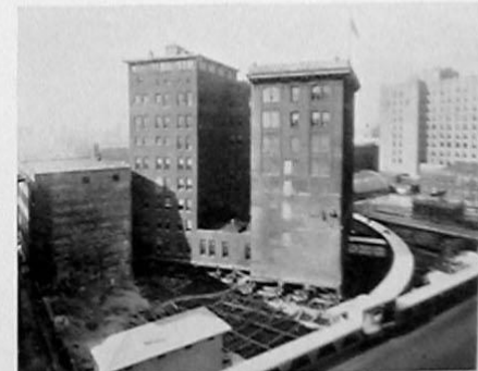
FIGURE 9. On November 1 the structure had moved around to the half-way point.
