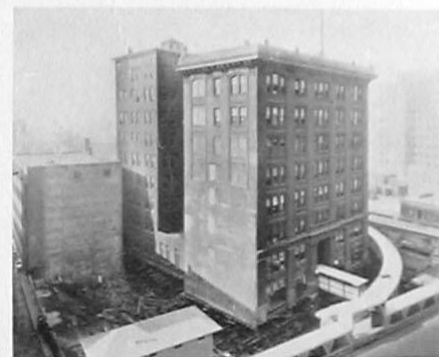
FIGURE 7. By October 28 the turn of the building was becoming quite apparent.
