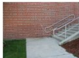
brick wall and stairs
