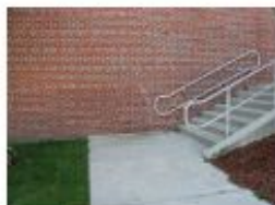
brick wall and stairs
