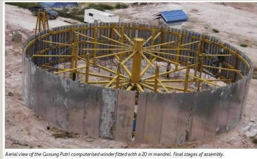
Aerial view of the Gunung Putri computerised winder fitted with a 20 m mandrel. Final stages of assembly.
