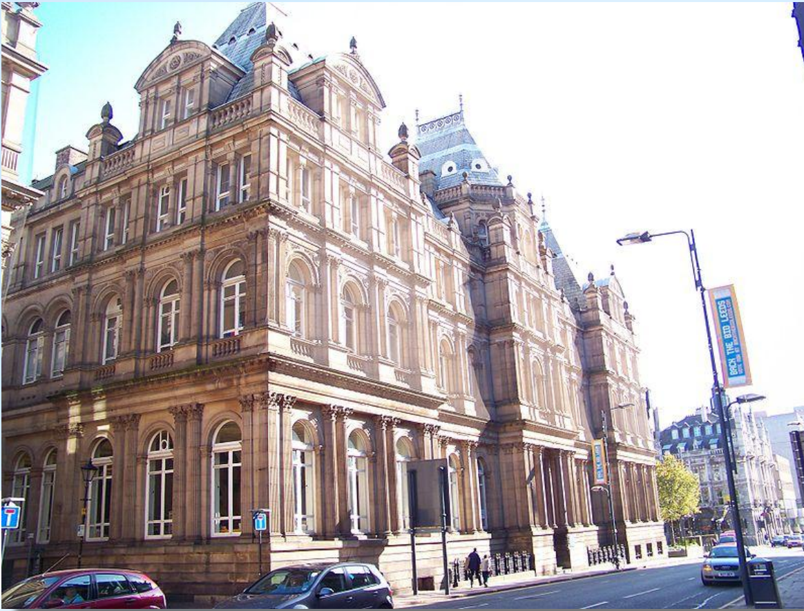
Leeds Central Library
