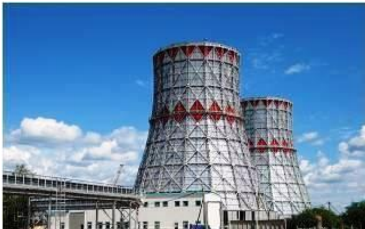
Tobolsk Heat and Power Generating Plant
