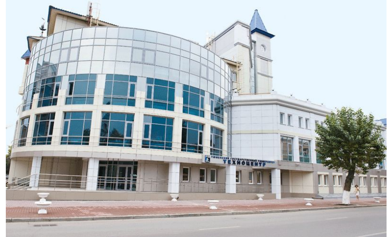
New building of Techno Park of Tyumen State University, Tyumen
