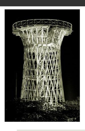
The round cone tower body consists of 6 sections with a height of 25 meters each.
