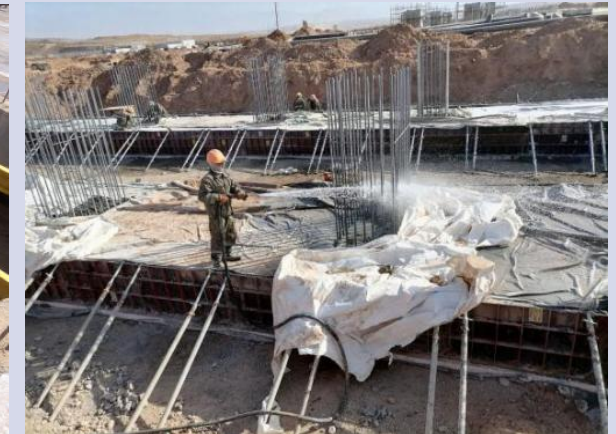
513-01 Gas engine generators building Concrete curing of foundation
