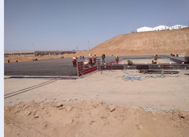
514-01 Mechanical and repair shop Installation of formwork on flooring monolithic areas
