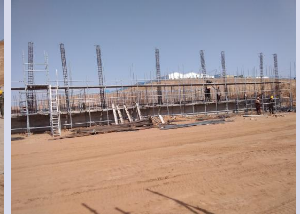
511-00 Main control room Reinforcement of wall columns
