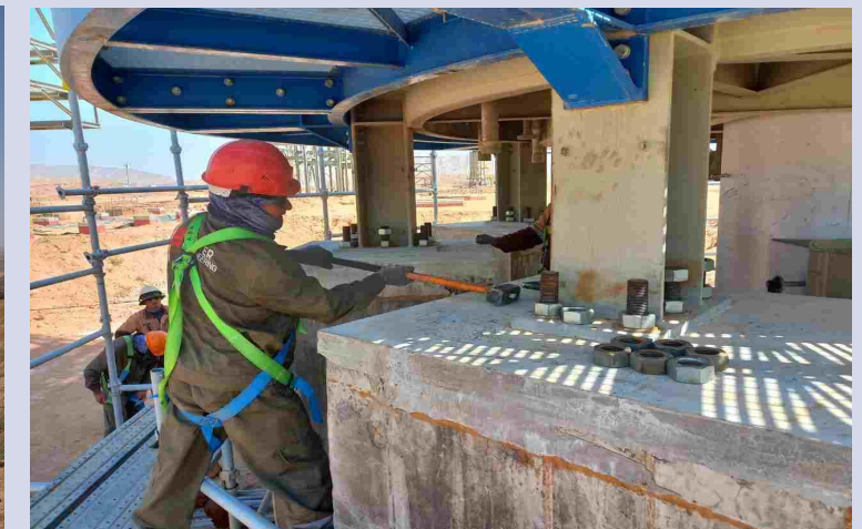
216-01-FA-01 Regeneration Gas Heater Bolts tightening
