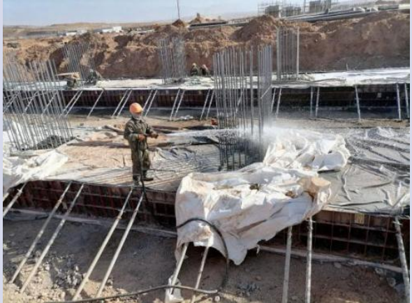
513-01 Gas engine generators building Concrete curing of foundation
