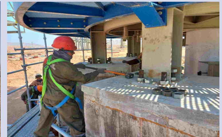
216-01-FA-01 Regeneration Gas Heater Bolts tightening
