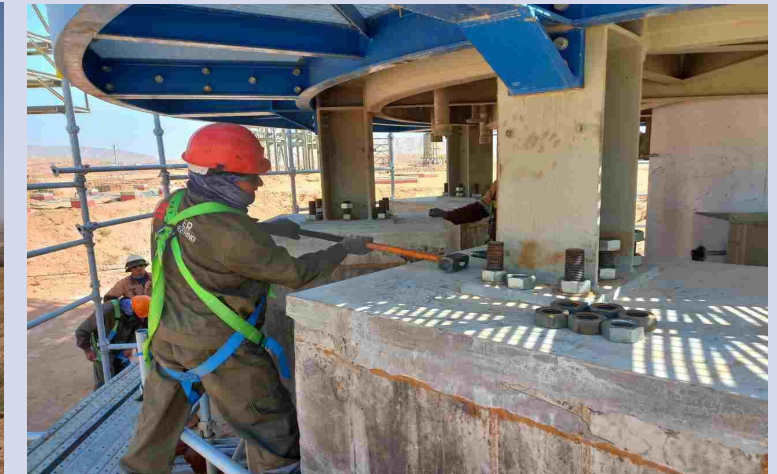
216-01-FA-01 Regeneration Gas Heater Bolts tightening
