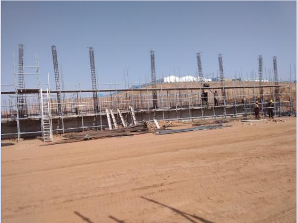
513-01 Gas engine generators building Concrete curing of foundation
