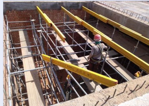
514-01 Mechanical and repair shop Installation of formwork on flooring monolithic areas
