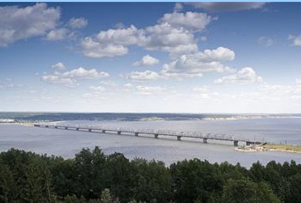
The bridge in Ulyanovsk is very long, about 3 km.
