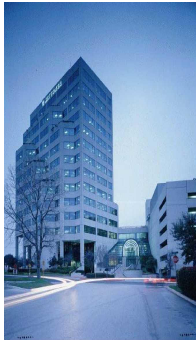
KCI Tower, San Antonio
