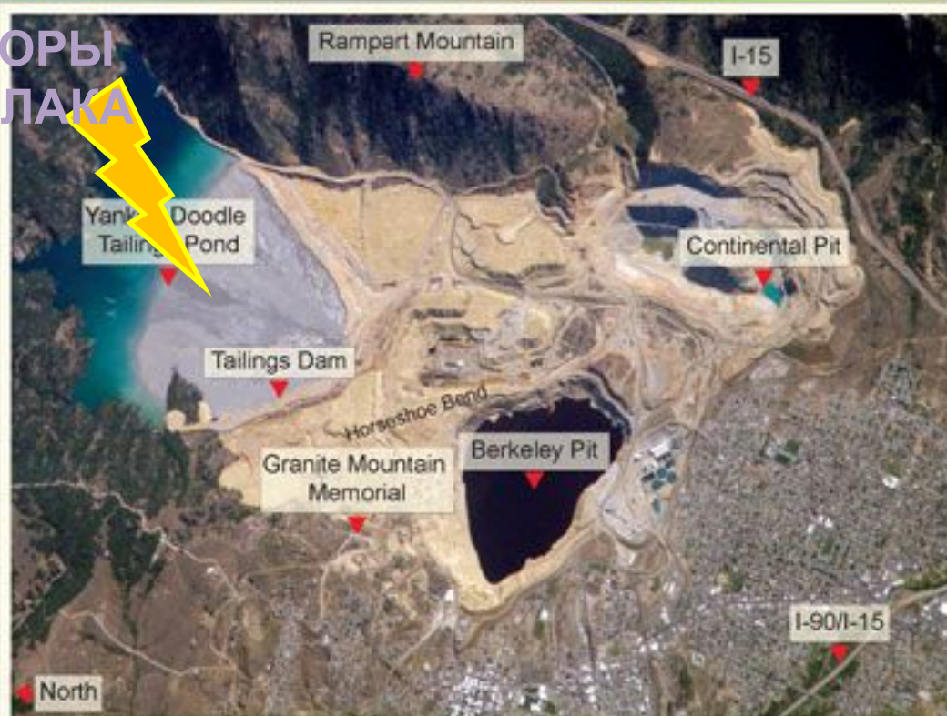
This 2006 photo from the NASA Earth Observatory shows the Berkeley Pit and the surrounding area after the construction of the Horseshoe Bend Water Treatment Plant and after the resumption of mining at the Continental Pit.
