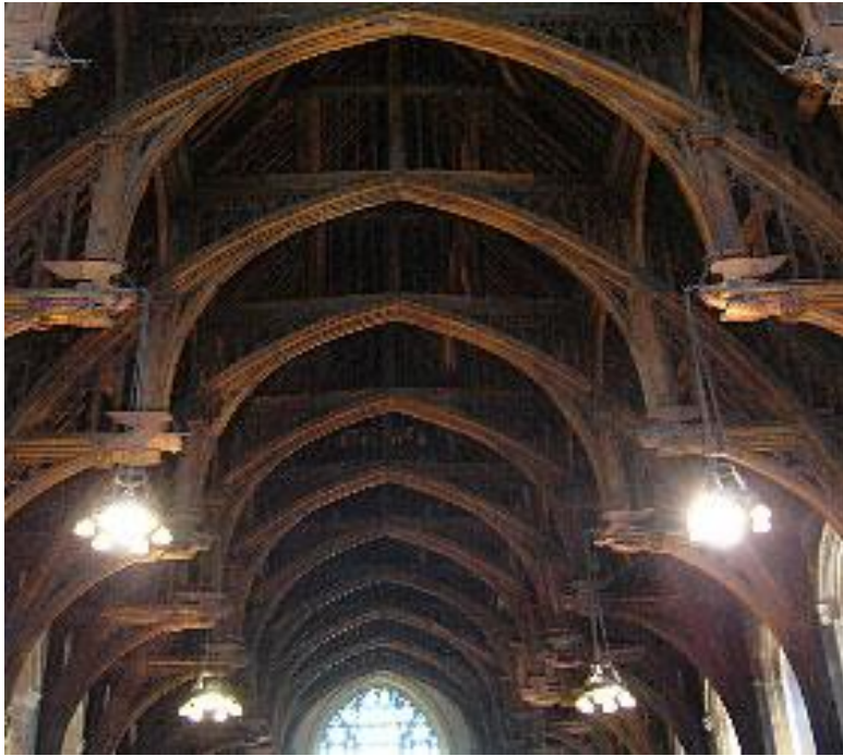
The medieval wooden ceiling of Westminster Hall (which survived the 1834 fire)
