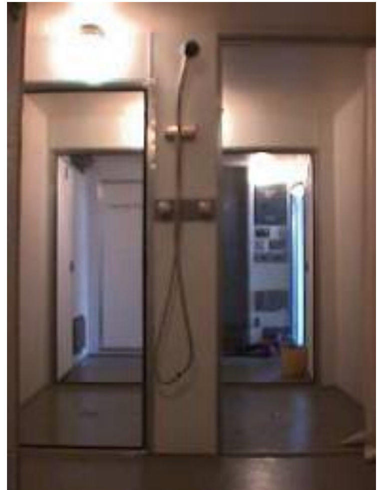
Emergency Response Decon Unit Union County, NJ
