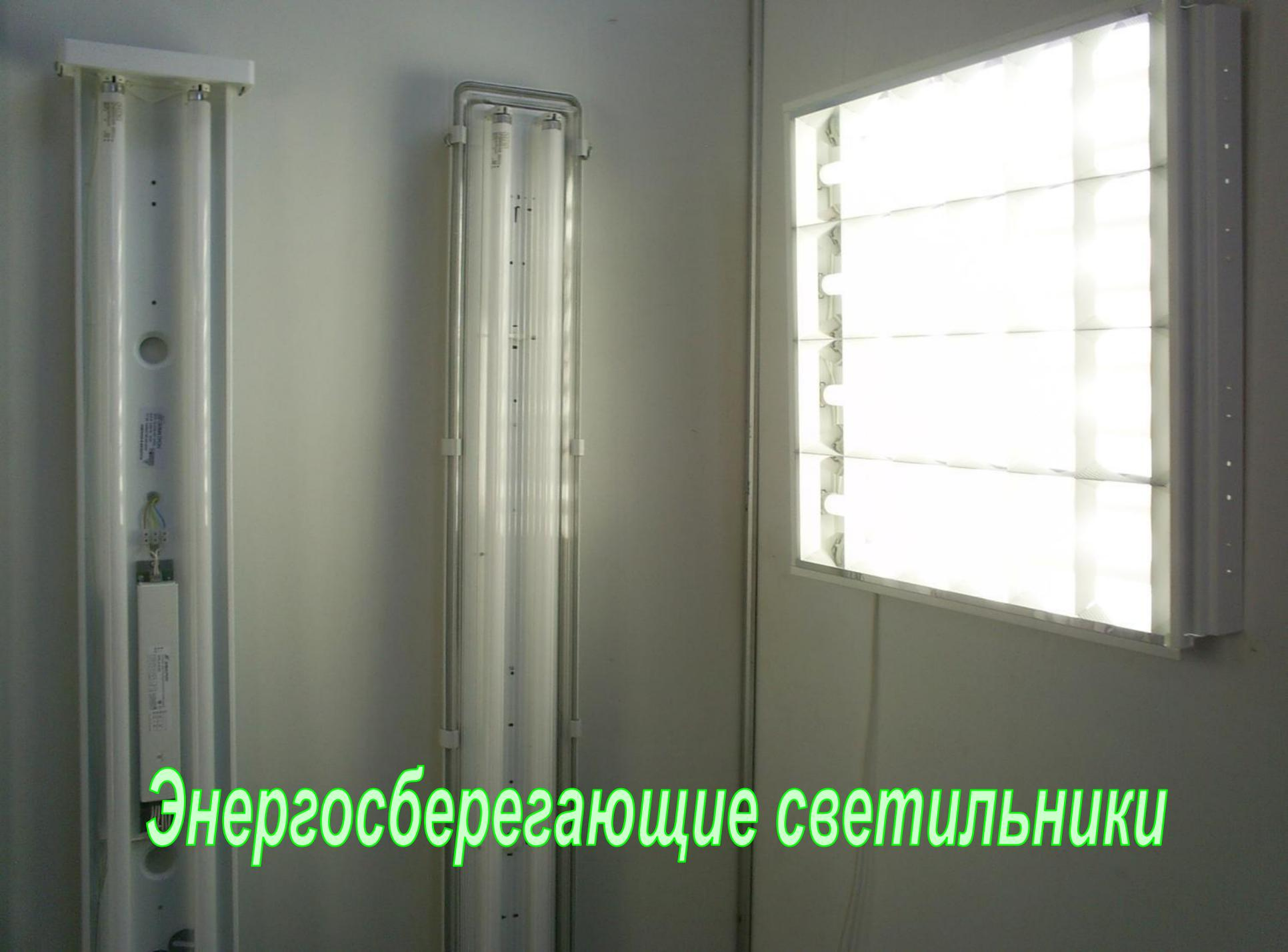
The image shows three energy-saving lighting fixtures. On the left and in the center are two long, vertical fluorescent-style fixtures with their outer covers removed, revealing the internal tubes and ballasts. On the right is a rectangular, recessed ceiling light fixture with a grid pattern, which is illuminated and glowing. The background is a plain, light-colored wall.
