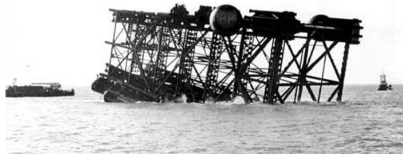
BP Forties platform lamellar tears were produced when attempting the repair of lack of root penetration in a brace weld
