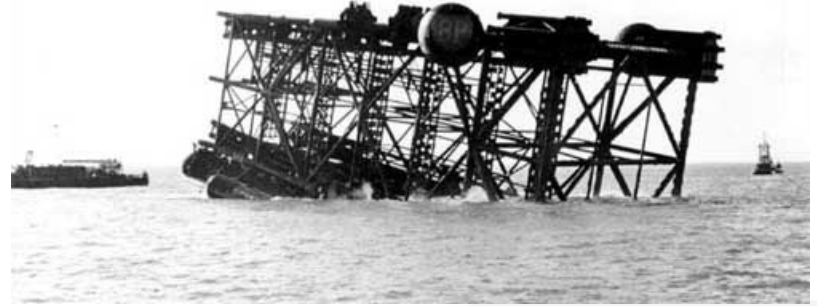
BP Forties platform lamellar tears were produced when attempting the repair of lack of root penetration in a brace weld
