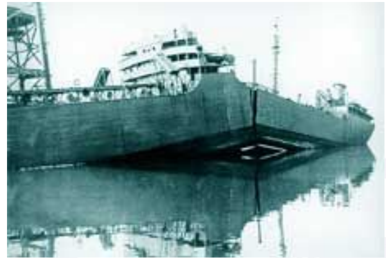
The SS Schenectady, an all welded tanker, broke in two whilst lying in dock in 1943. Principal causes of this failure were poor design and bad workmanship
