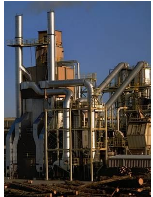
Scrubber at work
