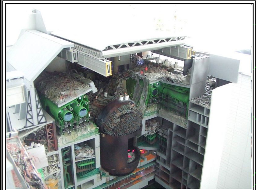
Model of Chernobyl reactor after the lid of the reactor chamber blew off. Chernobyl Museum, Kiev, Ukraine.
