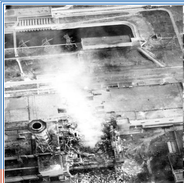
Aerial view of the damaged core on May 3, 1986. Roof of the turbine hall is damaged (image center). Roof of the adjacent reactor 3 (image lower left) shows minor fire damage.
