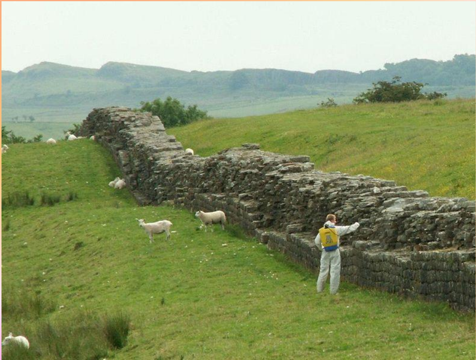
Hadrian's Wall near Birdoswald Fort, with man spraying weed-killer to reduce biological weathering to the stones
