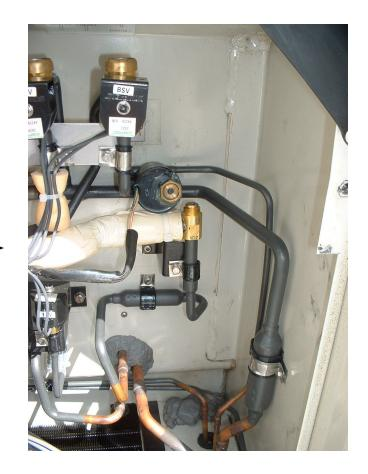
Step 2-3 Put emergency coil cap on valve body
