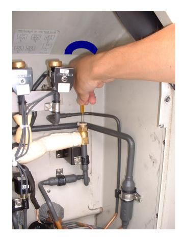
Step 2-5 Slightly open ( 60°) with counterclockwise direction
