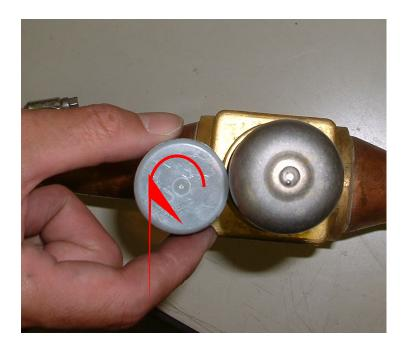
\*Emergency magnet is in onboard spare parts kit
