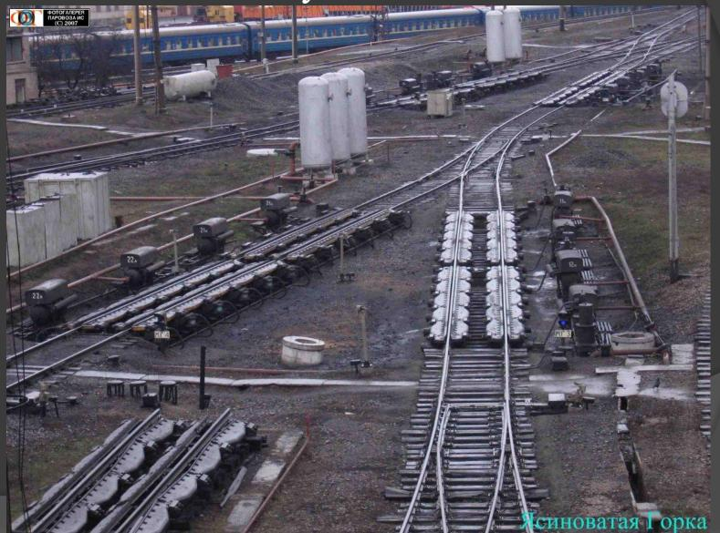
A hump yard in which wagons are propelled over a hump to run down a steep slope into sorting sidings
