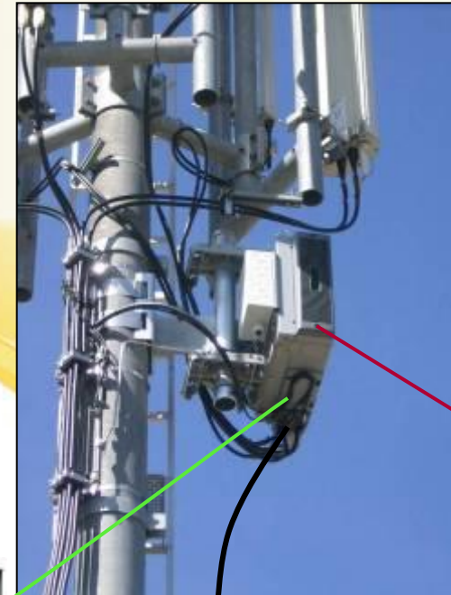
Power cable directly connected to DCDB
