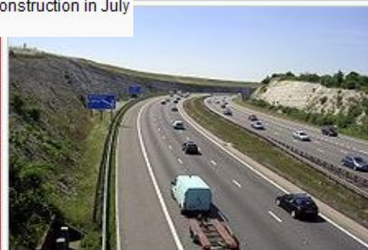
The Twyford Down cutting in August 2005
