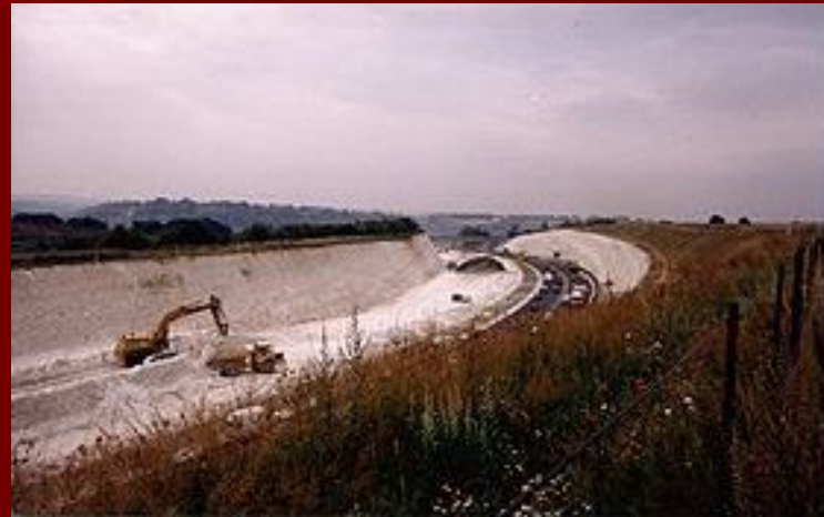
Twyford Down cutting during M3 construction in July 1994
