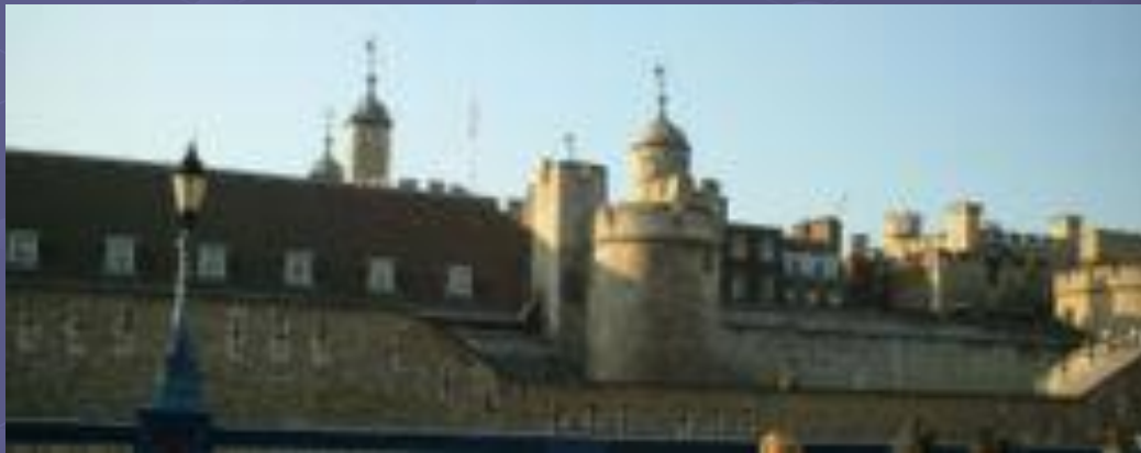
The Battlements, as seen from Tower Bridge approach
