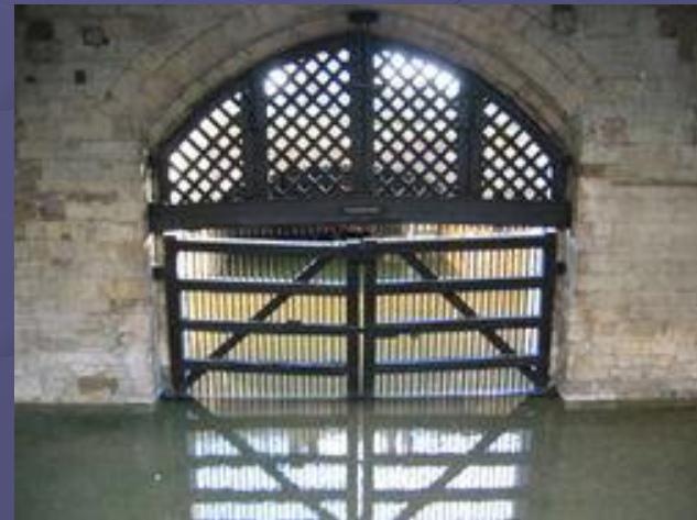
The Traitors' Gate
