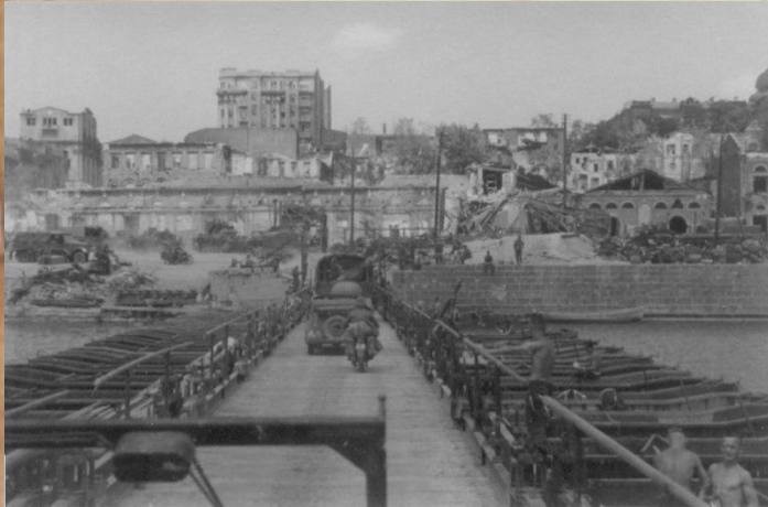
Temporary bridge across the river Don, 1942, March
