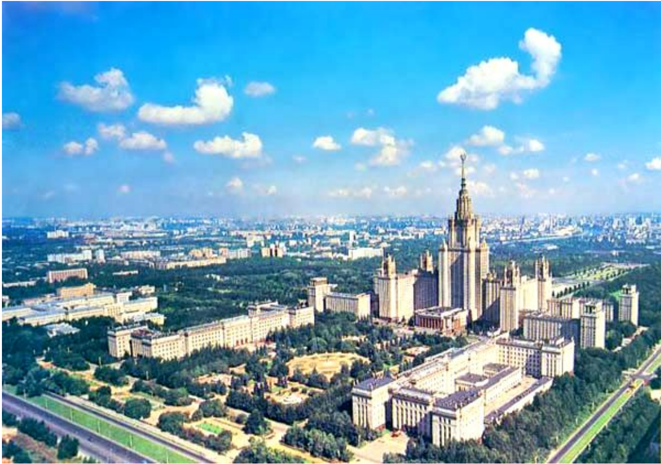
Today's 31-stored Main Building on the Sparrow Hills
