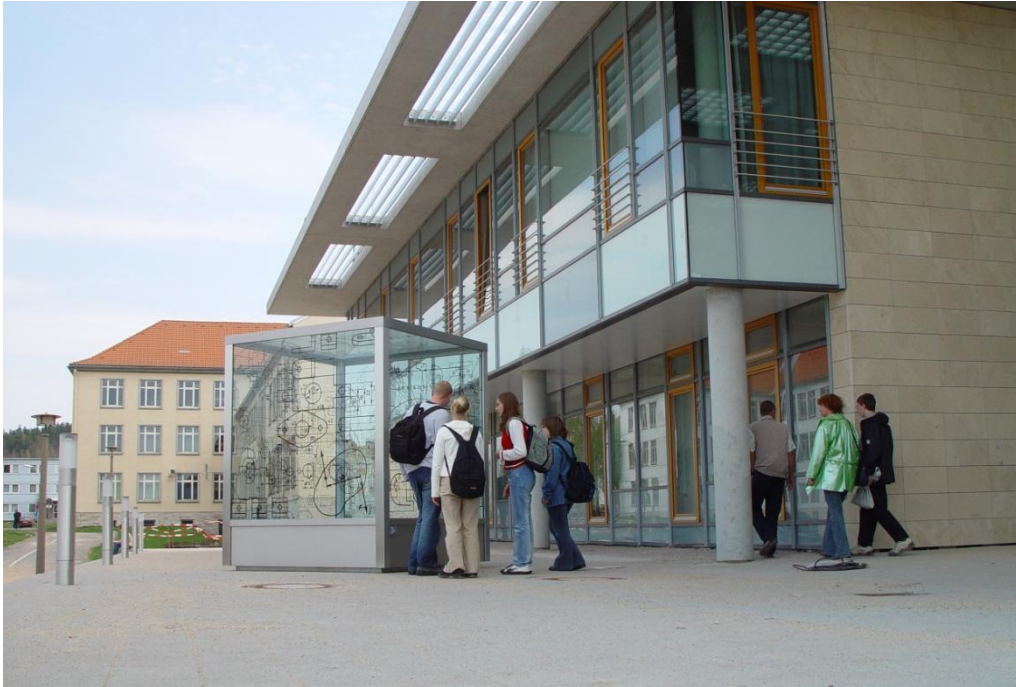
Newtonbau (Building for Department of Mechanical Engineering)
