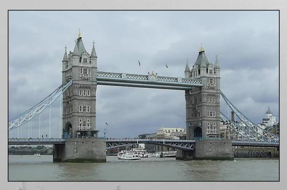
Jones' engineer, Sir John Wolfe Barry devised the idea of a bascule bridge 800 feet in length with two towers each 213 feet (65 m) high, built on piers. The central span of 200 feet (61 m) between the towers was split into two equal bascules or leaves, which could be raised to an angle of 83 degrees to allow river traffic to pass.
