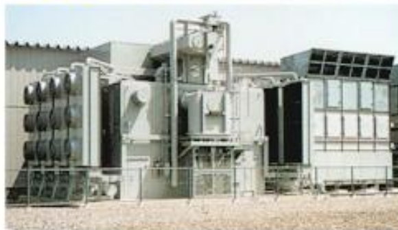
↓ Converter transformer
