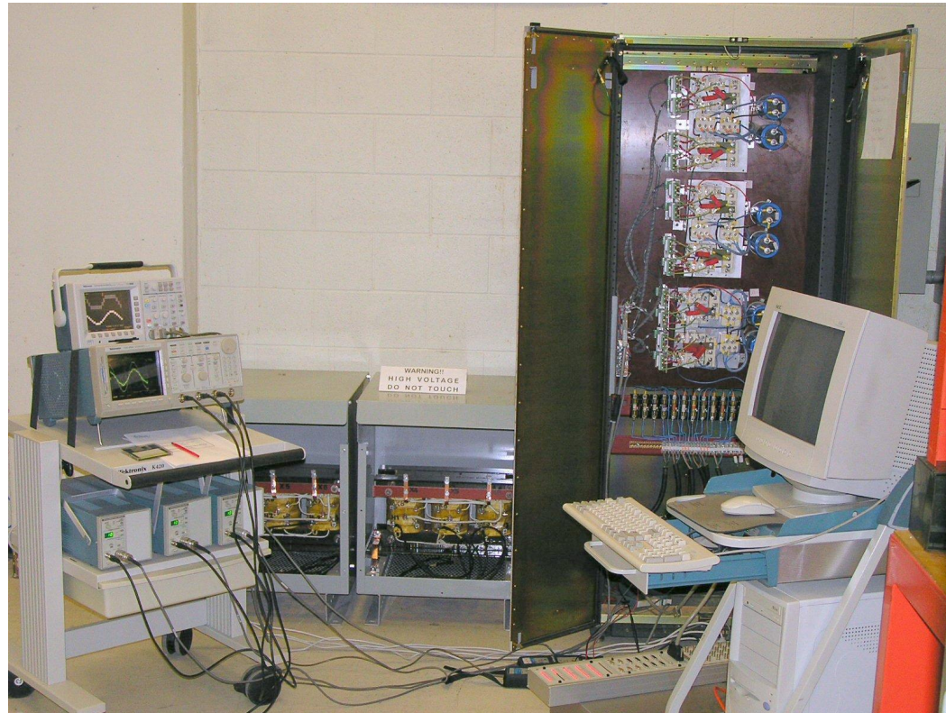
Five-Level NPC/H-Bridge Inverter System with dual 18-pulse rectifier LEDAR, Ryerson University
