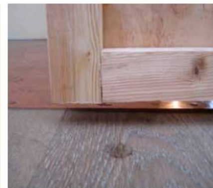
Ensure the panels are hanging just off the floor of the window
