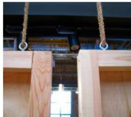
Hang panels one by one before attaching together. See page 2 for how to knot rope
