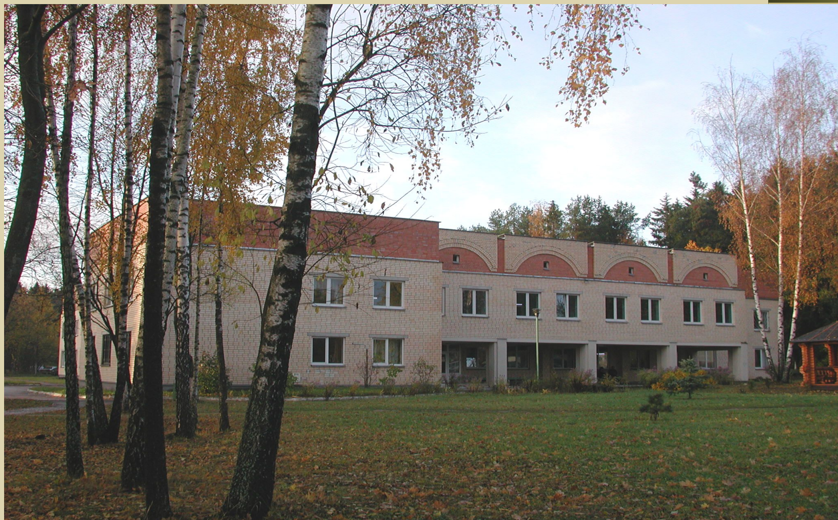
Modernized building for oncological mammalogical department
