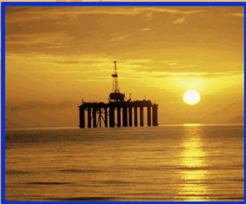
Site Automation and Control
