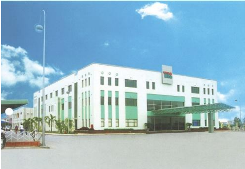
Techno Center, Thang Long Industrial Park
