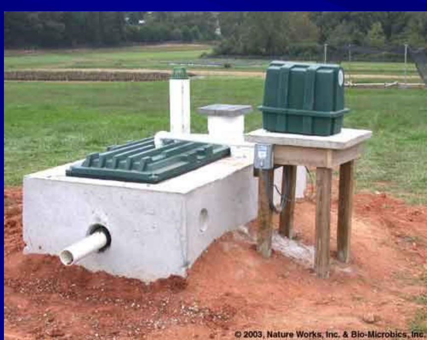
© 2003, Nature Works, Inc. & Bio-Microbics, Inc.
