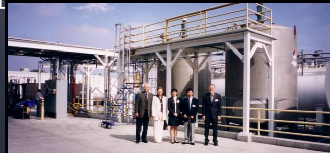
Manufacturing plant, San Jose, CA
