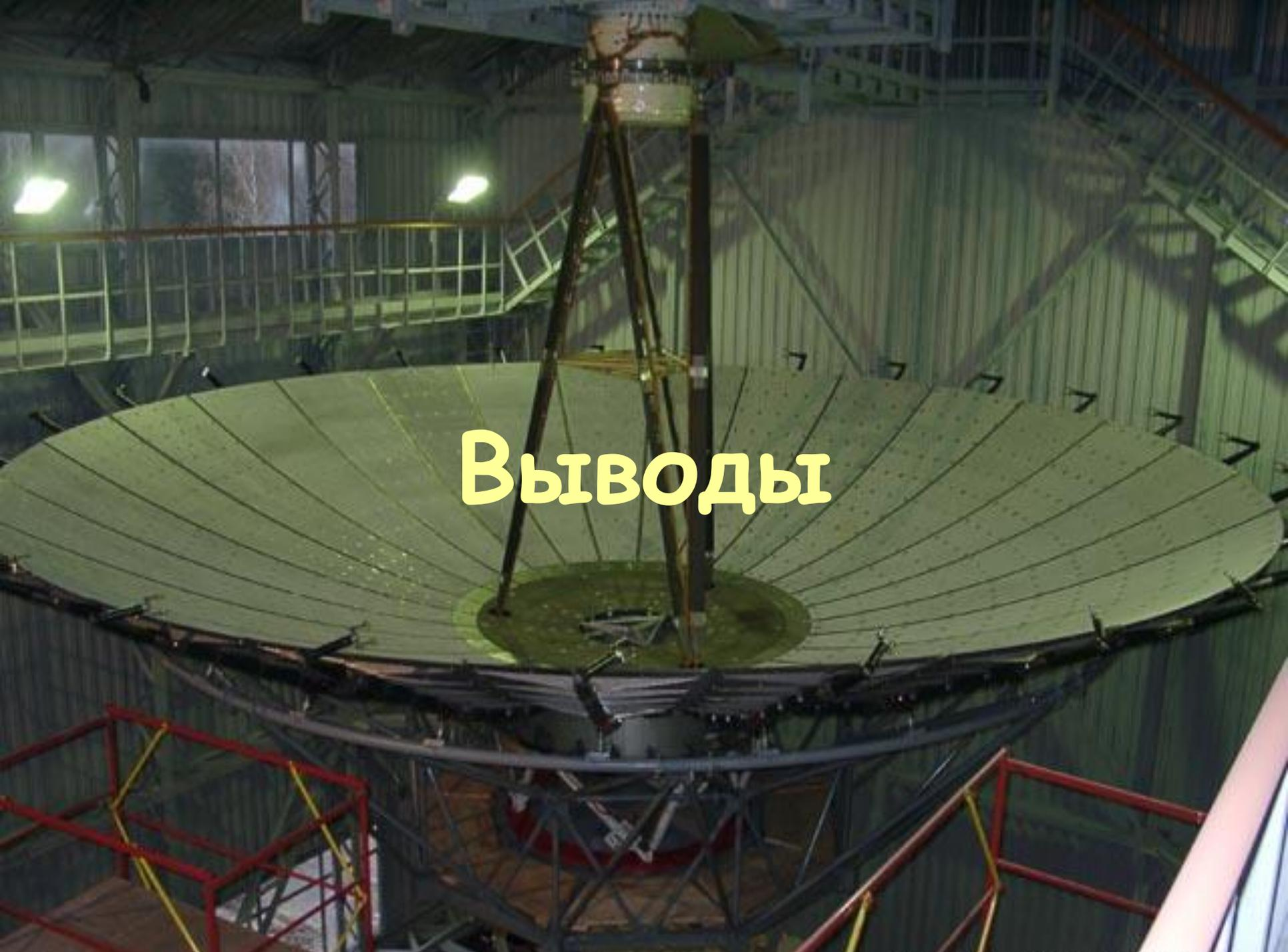
A large parabolic satellite dish antenna is shown inside a building. The dish is made of many small panels and is mounted on a complex metal structure. A central mast with a receiver is positioned at the focus of the dish. The building has a corrugated metal interior wall and a walkway with railings is visible in the background. The word "Выводы" (Conclusions) is written in large yellow Cyrillic letters across the center of the dish.
