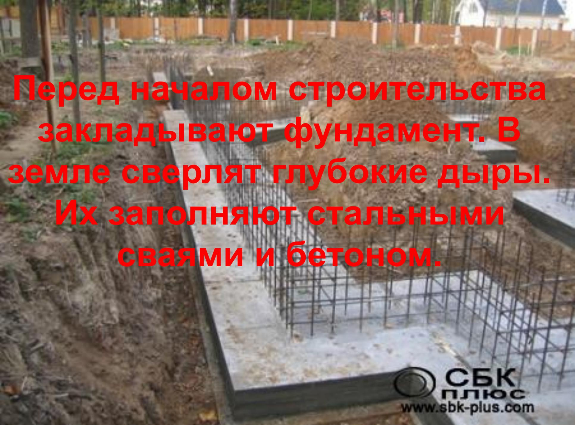
A photograph of a construction site showing the foundation stage. Several rectangular concrete pits have been dug into the ground. Inside each pit, a cage of steel reinforcement bars (rebar) is visible, ready for a concrete pour. The ground around the pits is uneven and appears to be recently excavated. In the background, there is a wooden fence and some trees. The text is overlaid in large, bold, red letters.
